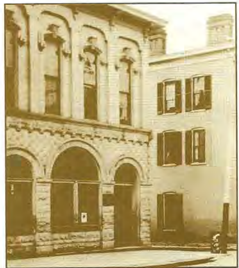
Bank of Shelbyville and Armstrong Hotel South Side of 6th & Main Street 1909
